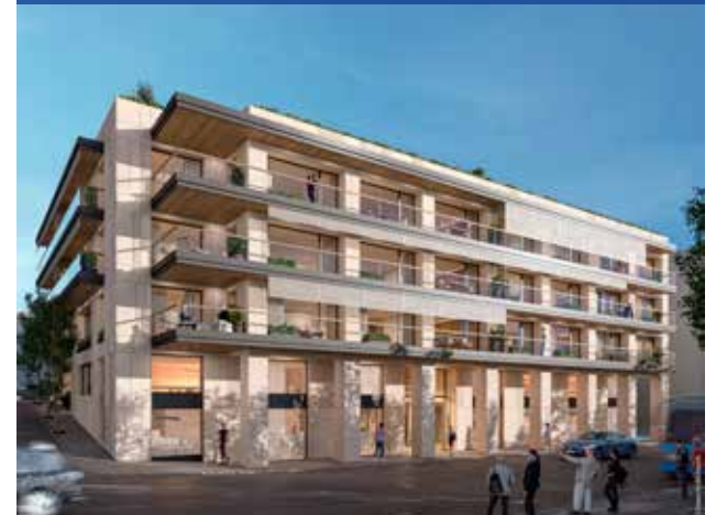
Mets Residential and Office Building
